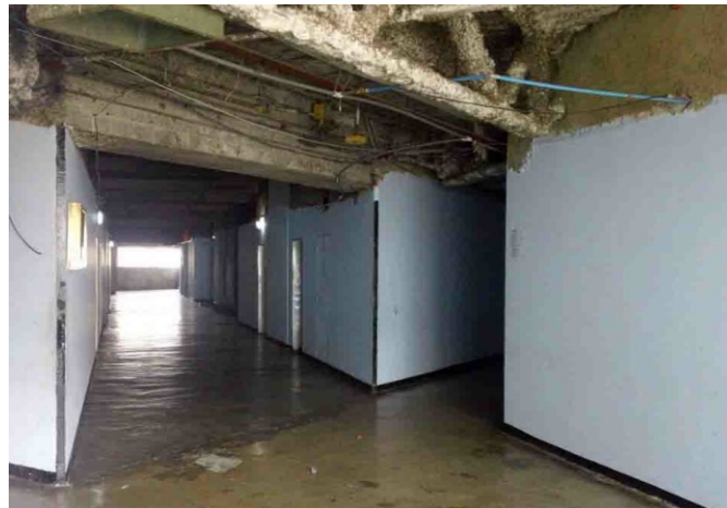
Fig. 4. Interior corridors of Torre David
