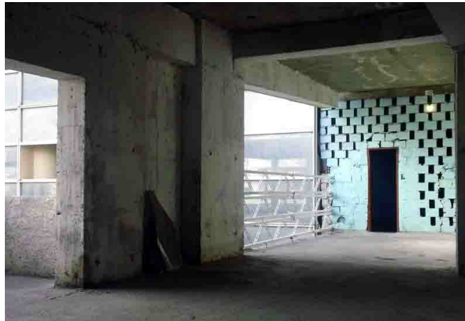
Fig. 3. The building was designed as an office tower, for the present residential use, the dimensions of services and circulation areas is disproportionate.
