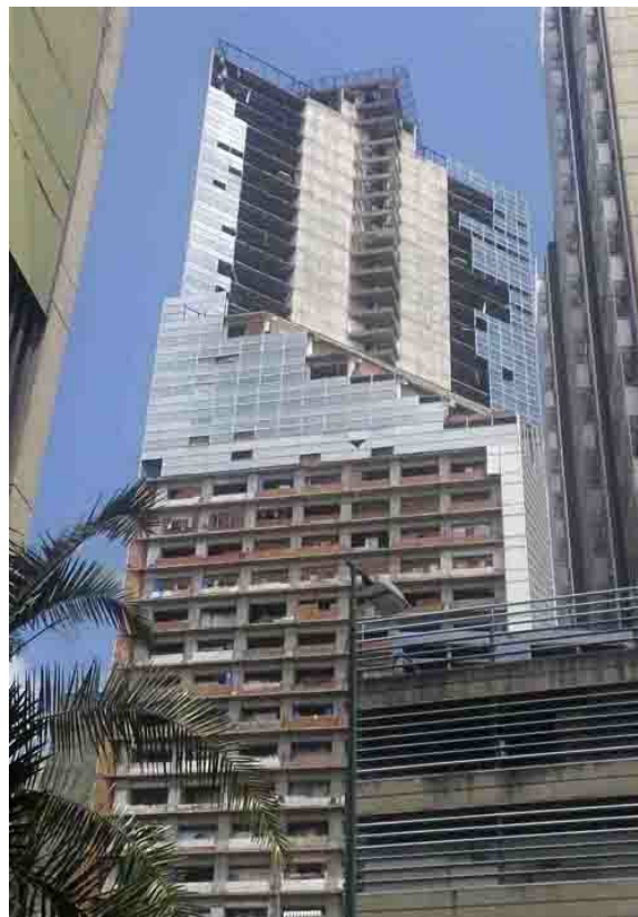
Fig. 2. Exterior view of the Torre David in Caracas.
